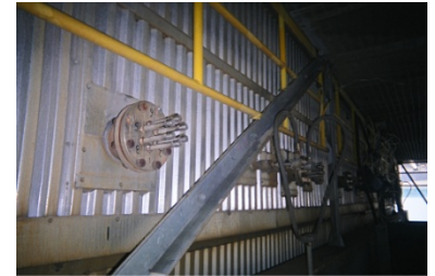
AIG Tuning Grid Sampling Ports
